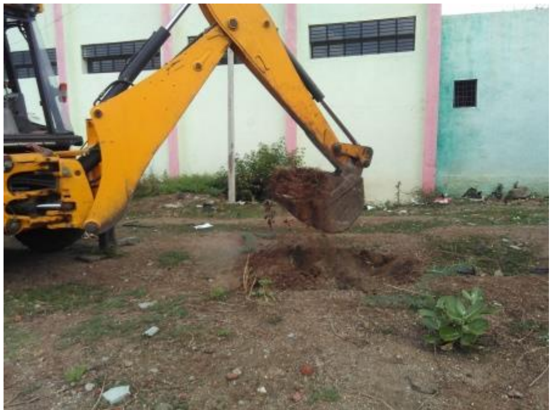
Digging for tree plantation in SGP Campus.
